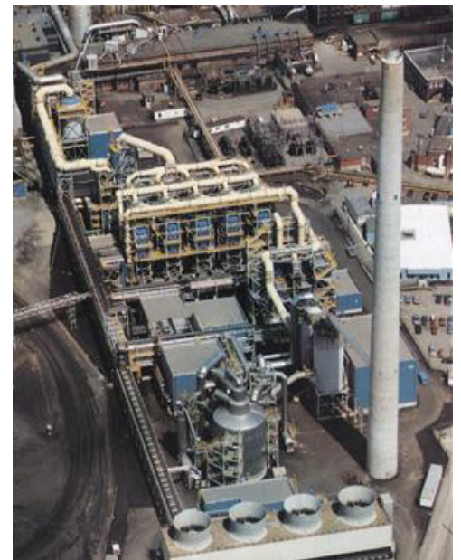
The smelter for sulfide ores produces sulfur dioxide gas. This is scrubbed from the flue gases to make sulphuric acid for leaching copper from oxide ores. Scrubbing sulfur dioxide also protects the environment. (Courtesy of Xstrata.)
